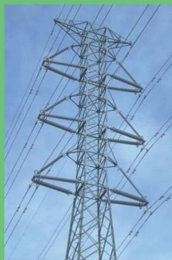
Fig. 2: Rigid cross-arm solution using braced line post concept with double V-posts (245 kV).
